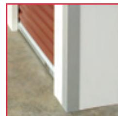
Corawall Hall Partition is an alternative to corrugated securewall, these 12" self-aligning panels interlock so that there are no exposed screws or edges except where attached at the top channel. Top and bottom channel included provides additional strength for supporting panels. An added insurance, the Protective Package is available to keep these walls dent and ding free once installed.
